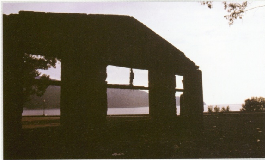
Burnt-out Italian facilities at Merkia.
