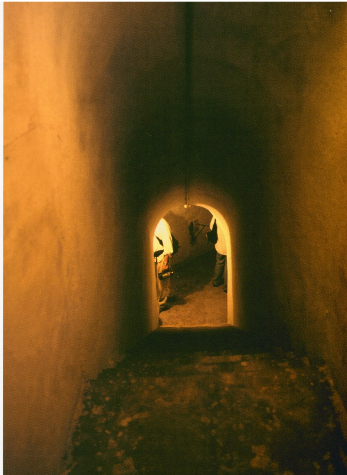
Inside the hospital: a corridor leading to another level in the heart of the mountain.
